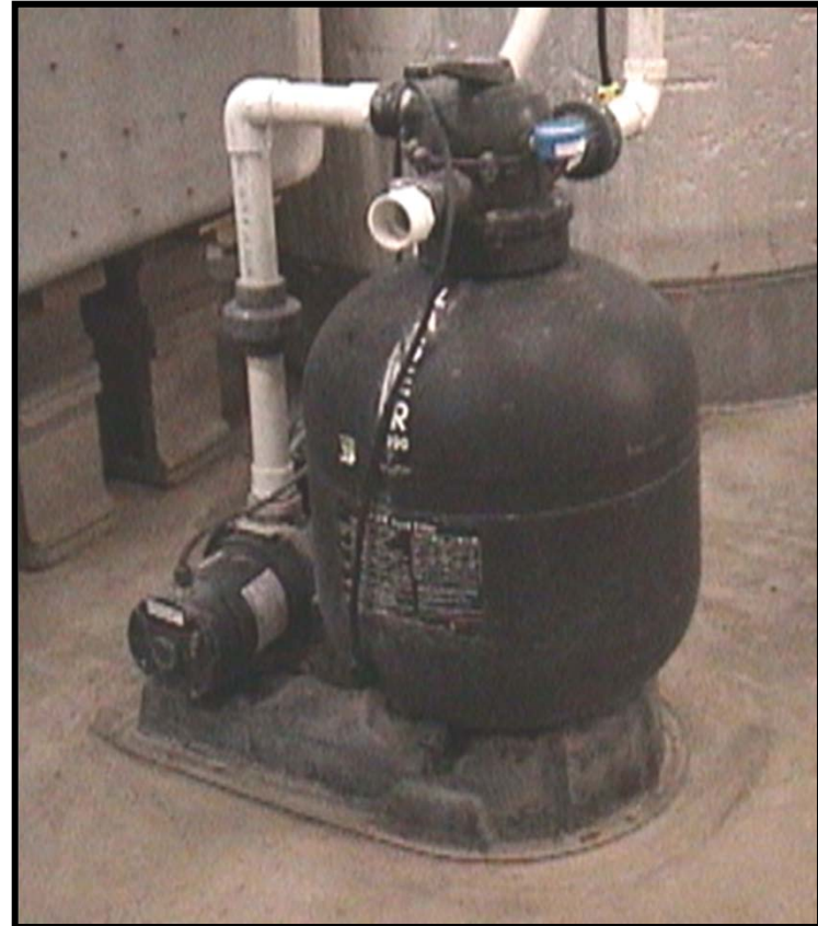
Pressurized downflow sand filter
